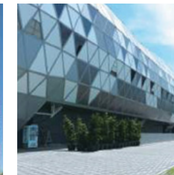
Kaohsiung Exhibition Center Kaohsiung, Taiwan
